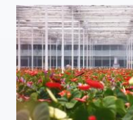
Central China Yanling Green House
